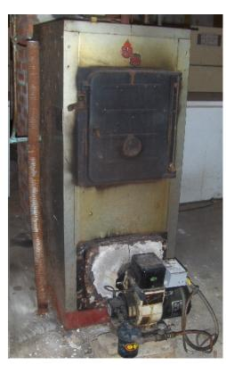
Since the street is supplied with gas, it is suggested that a gas fired burner be installed. This will eliminate the need for oil fuel deliveries and you can abandon the buried oil tank.
