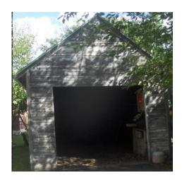
Our survey of the garage revealed that it is structurally damaged, crooked and leaning to the left. In an attempt to salvage the garage, we recommend the following corrections before the garage collapses and/or causes injury. It is believed that the condition of the garage may impact obtaining a FHA mortgage. Below is a survey
