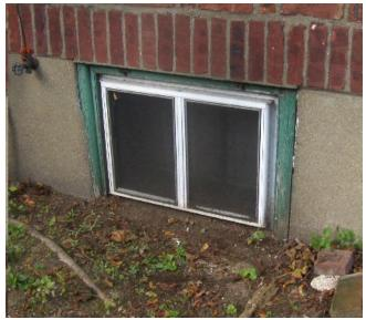
house to direct surface water away from the foundation. Before grading, install window wells and make sure the dirt is at least six inches below the level of the window sill.
